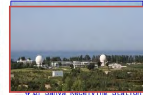
三亚站 Sanya Receiving Station
